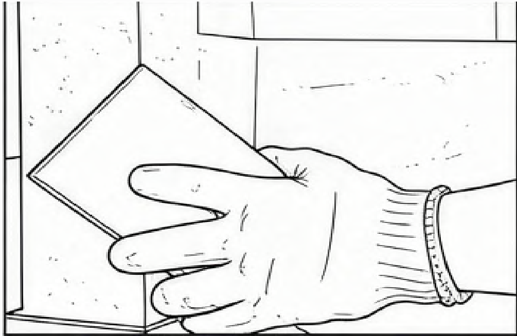
6. Sand the joints smooth and wipe the wall clean.
